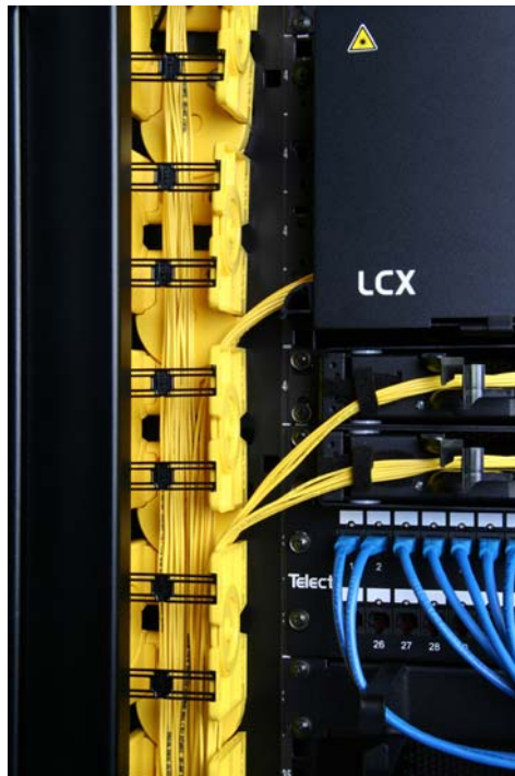
Top: 2" CableLinks, Telect part number 027-000-4200.
