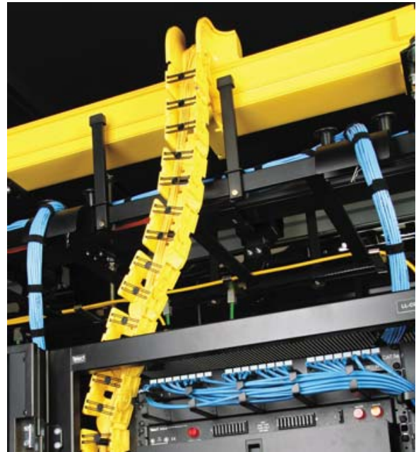
Figure 1 - CableLinks Assembly Installed
