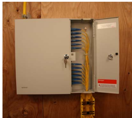
Figure 3: Each LANLINXS panel features two lockable doors for secure access to each side. Above, the panel is installed on a backboard. The provider side is closed and locked.
