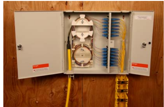
Figure 4: Fully configured Telect LANLINXS 24-port panel. Splice and storage is on the left-hand side of the panel, while patching takes place on the right. In this configuration, an incoming feeder cable enters at the bottom-left of the panel.
