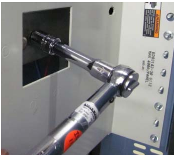
Figure 18 - Removing Hardware from the Distribution Panel
