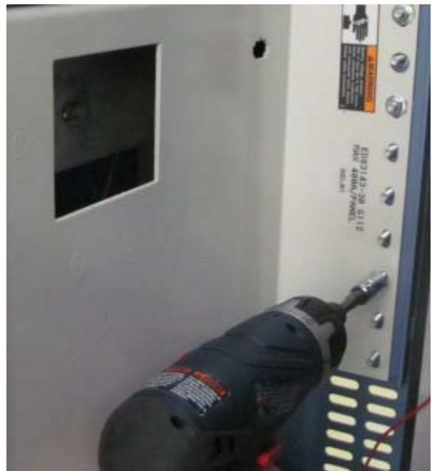
Figure 38 - Screwing in the Nuts at the Rear of the Distribution Panel
