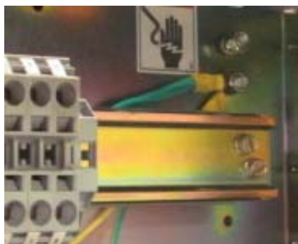
Figure 50 - Ground Lugs Connected to the Stud
