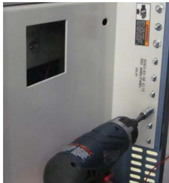
Figure 19 - Unscrewing the Nuts from the Rear of the Distribution Panel
