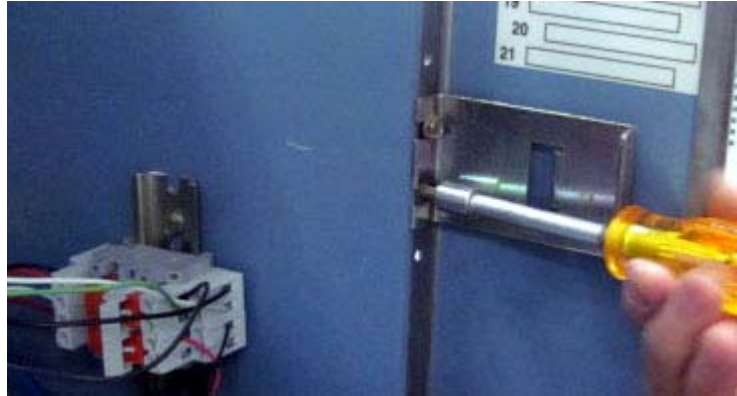
Figure 43 - Removing Bracket
