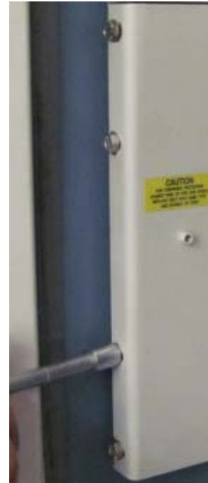
Figure 20 - Removing the Screws from the Side
