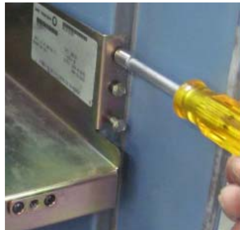
Figure 14 - Removing Screws from the Rectifier Shelf
