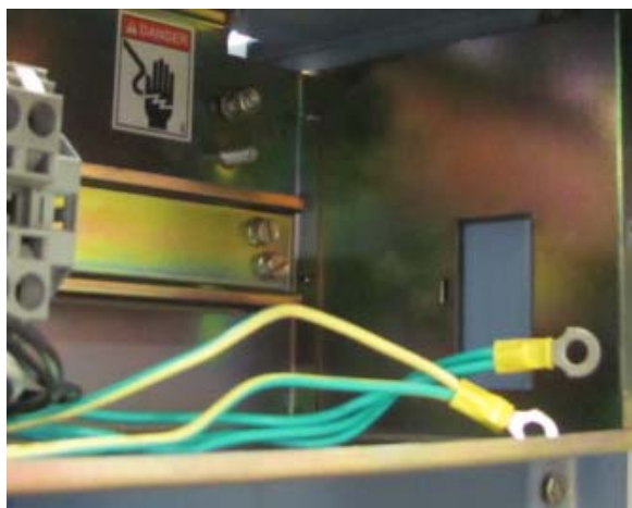
Figure 51 - Ground Lugs
