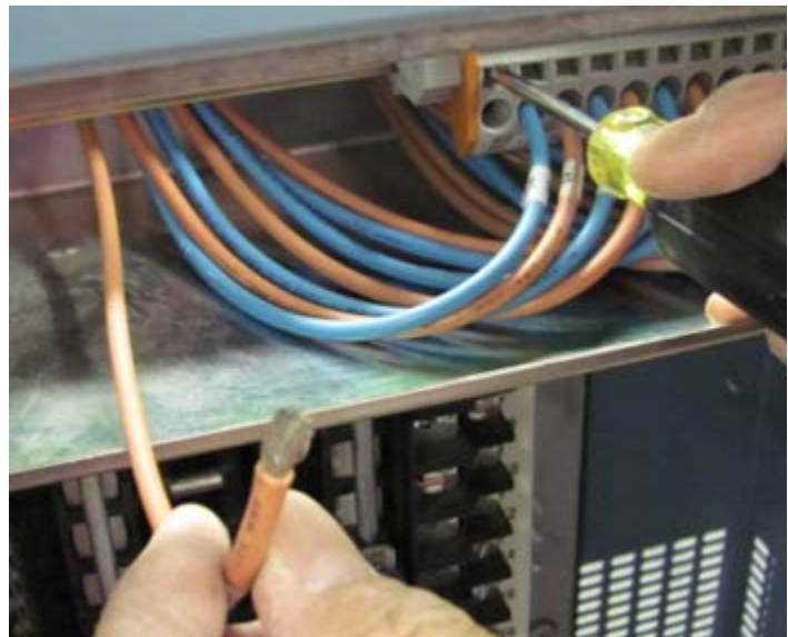
Figure 4 - Removing Rectifier's AC Wires
