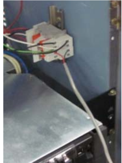
Figure 35 - Attaching the Relays to the Wall
