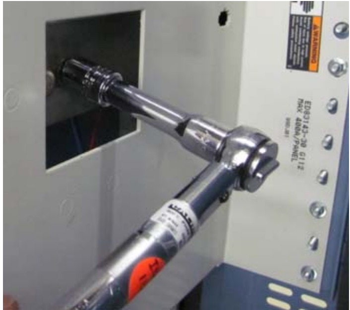
Figure 37 - Securing the Hardware to the Distribution Panel
