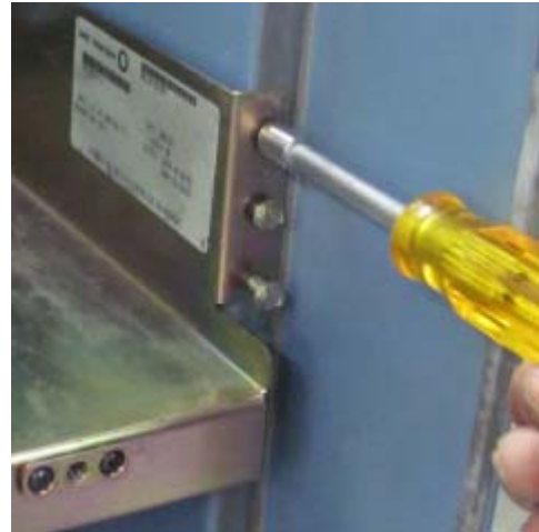
Figure 11 - Removing Screws from the Rectifier Shelf
